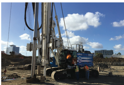
Condon-Johnson & Associates, Inc. installs drilled shaft foundations for a 6-level parking structure using the new Soilmec SR-95.
