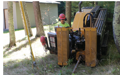
Michels Communications crew uses horizontal directional drilling while converting an overhead electrical system to an underground one.
